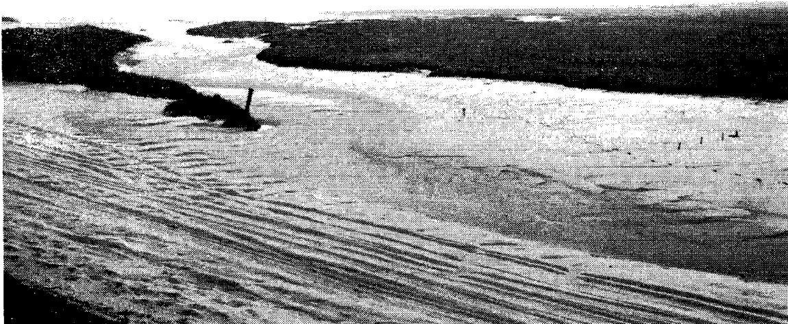
Fig. 10. Sand channels cut through the high marsh by vehicles allow for rapid movement of sand landward, accelerating the rate of infilling of Hatches Harbor.
