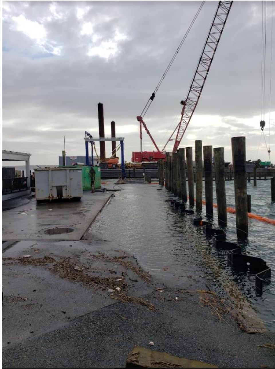
The North Wharf under construction, January 2024
