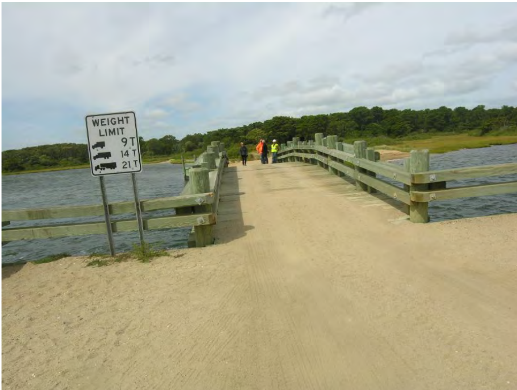
Photo 2: East at bridge weight posting sign.
