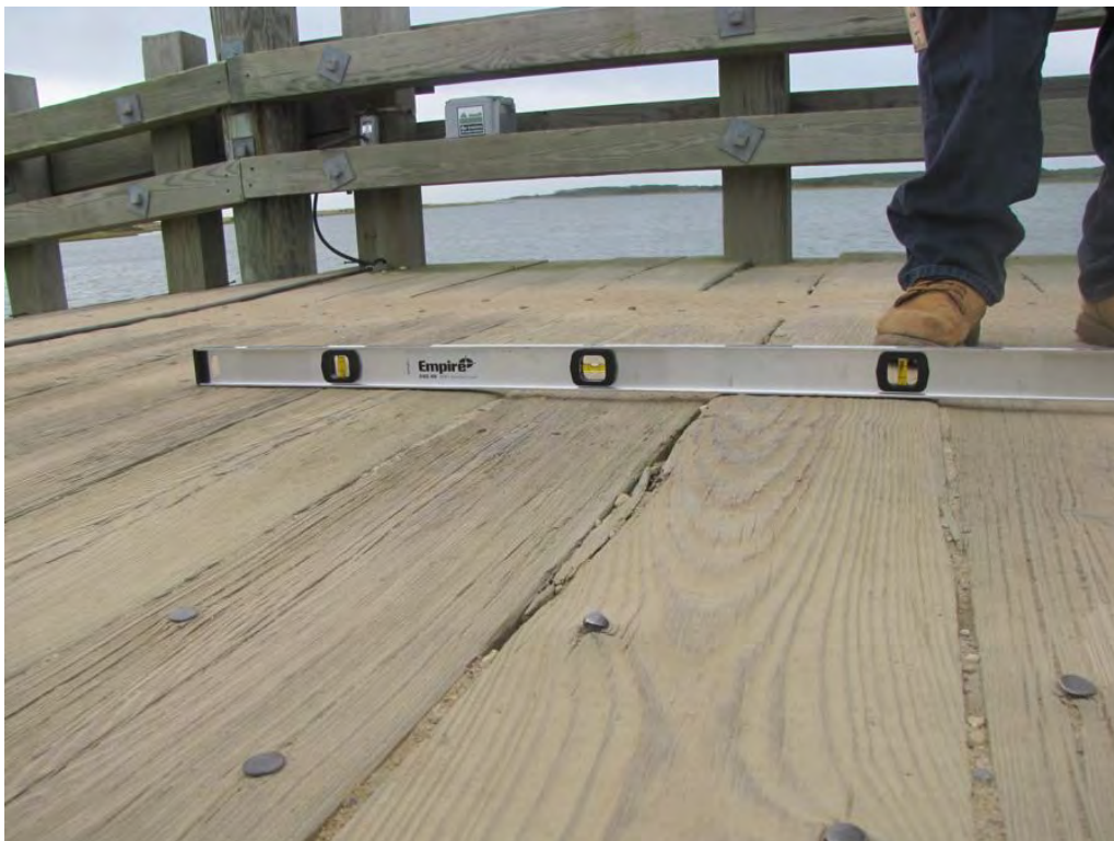
Photo 4: Typical washing boarding
