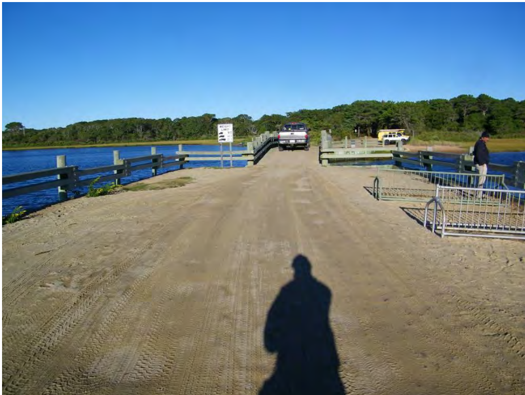
Photo 4: View east approach at bridge posting sign.
