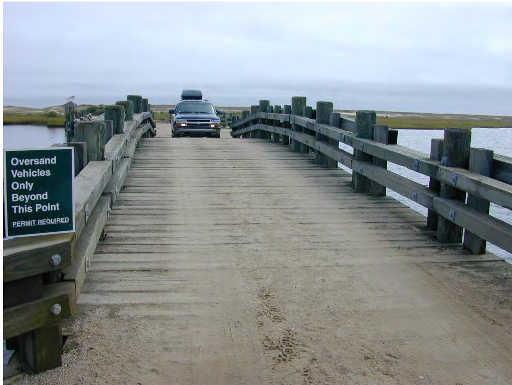
Photo 1: Build up of sand on wearing surface, minor settlement and rutting at both approaches
