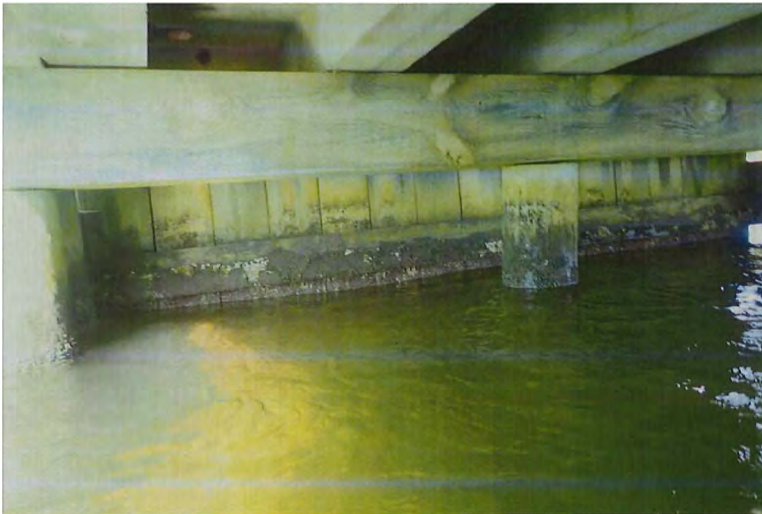
Photo 13: General view of west abutment bent & bulkhead, mildew staining & marine growth throughout.
