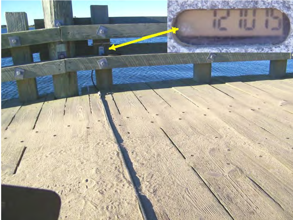
Photo 5: General view wearing surface and A.D.T. meter.
