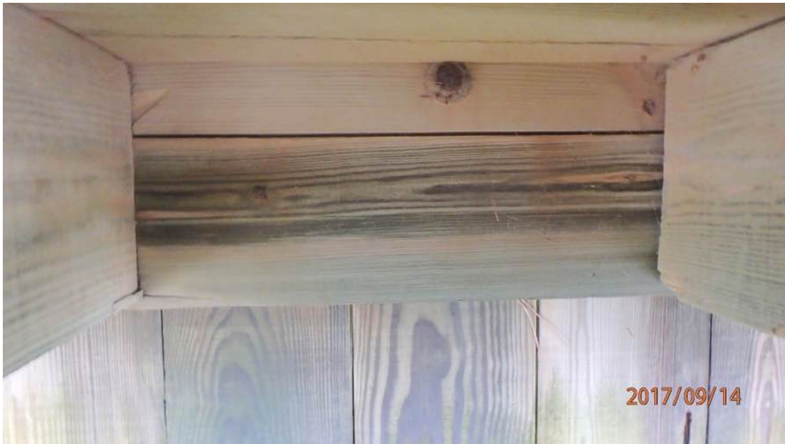
Photo 10: View timber backwall.
