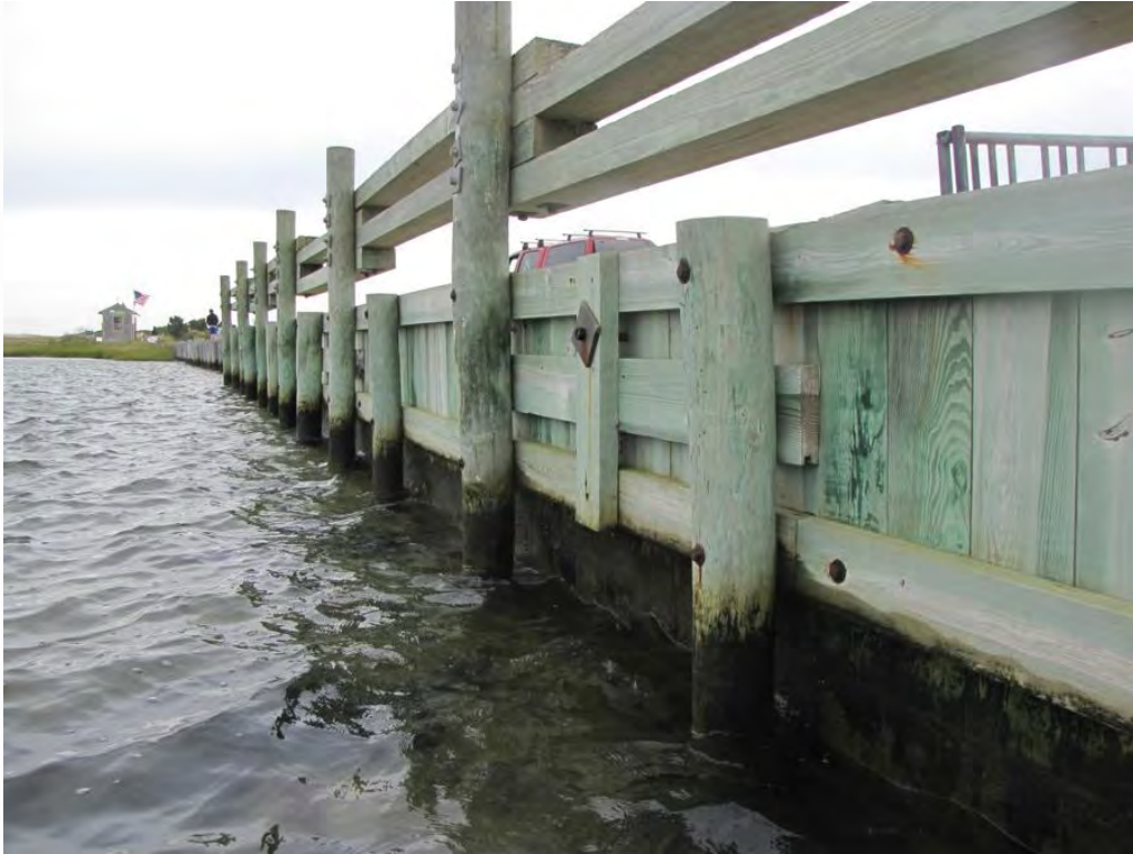
Photo 15: Typical wingwall and fasteners
