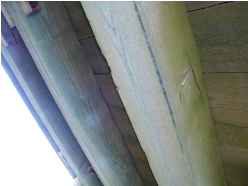
Photo 8: Typical underside of deck condition.
