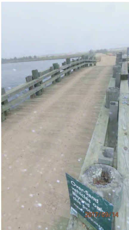
Photo 4: Looking east, general wearing surface condition.
