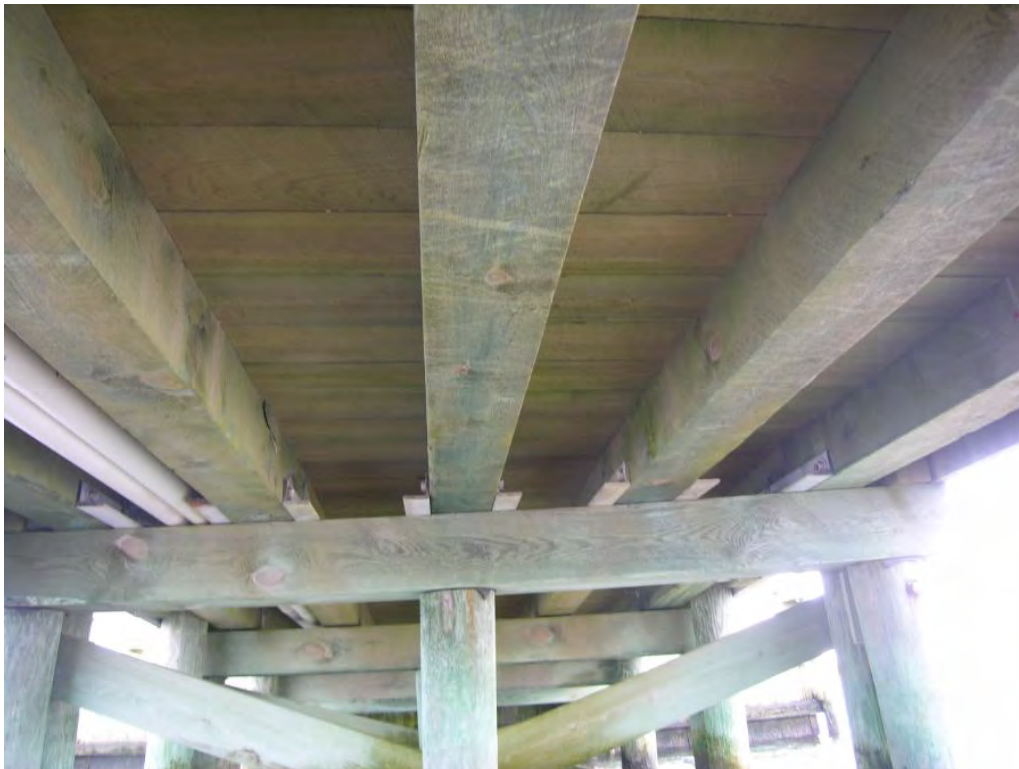
Photo 6: General underside main span.
