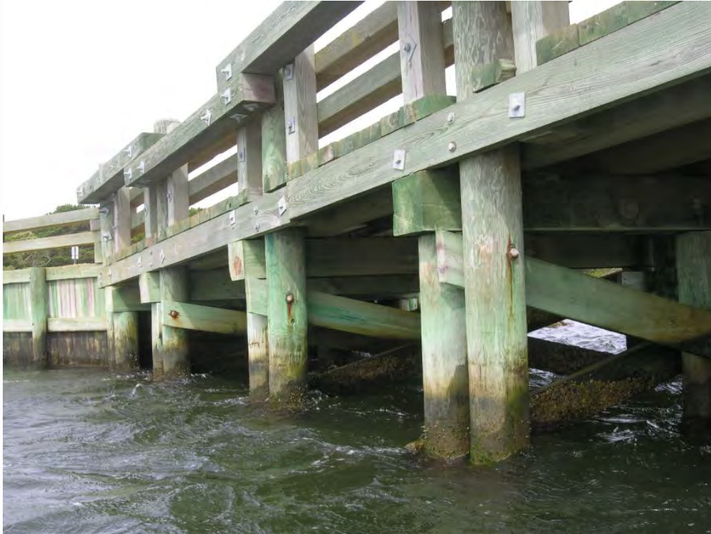
Photo 7: Southwest pile bents.
