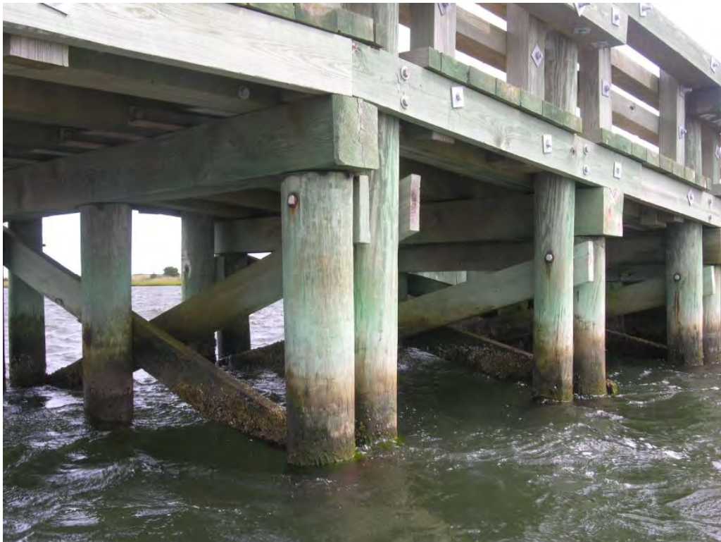
Photo 8: Southeast pile bents.
