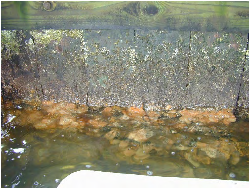
Photo 2: Build up of marine growth along both breastwalls
