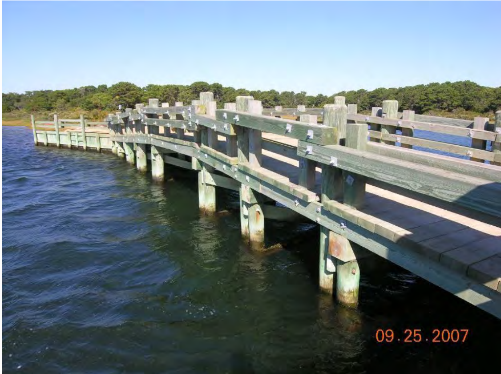
Photo 3: South elevation looking west
