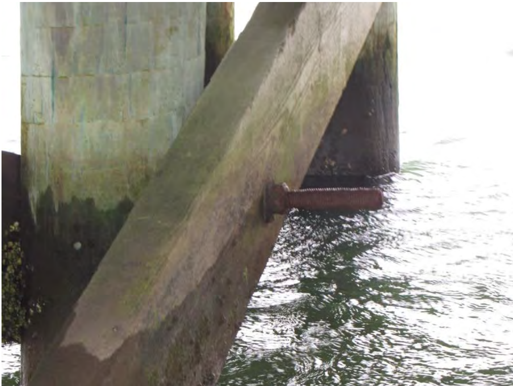
Photo 20: Isolated bolt starting to neck near nut
