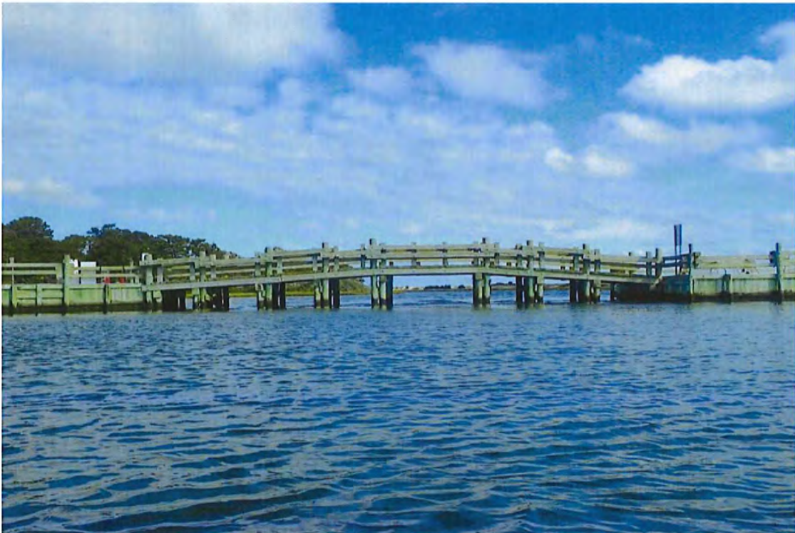
Photo 12: South elevation, typical vertical alignment of spans.
