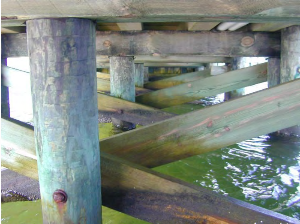
Photo 1: West view of pile bents from channel.
