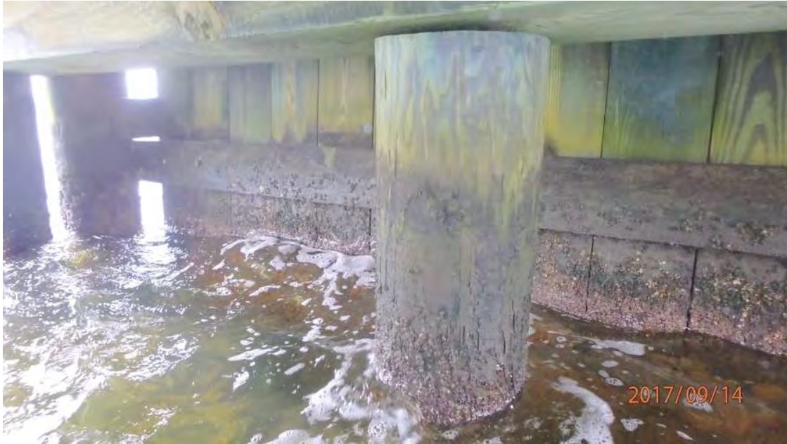
Photo 9: View west breastwall and pier 1 center column.
