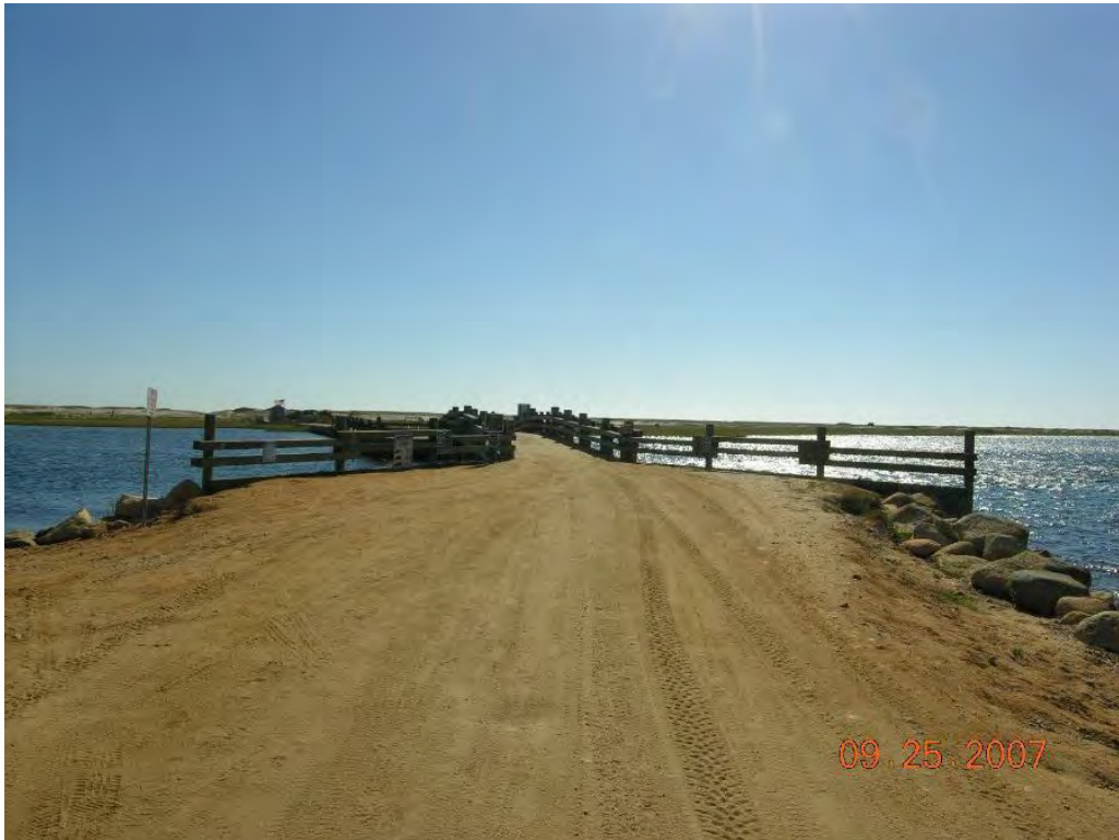
Photo 1: West approach showing weight posting sign on left approach rail
