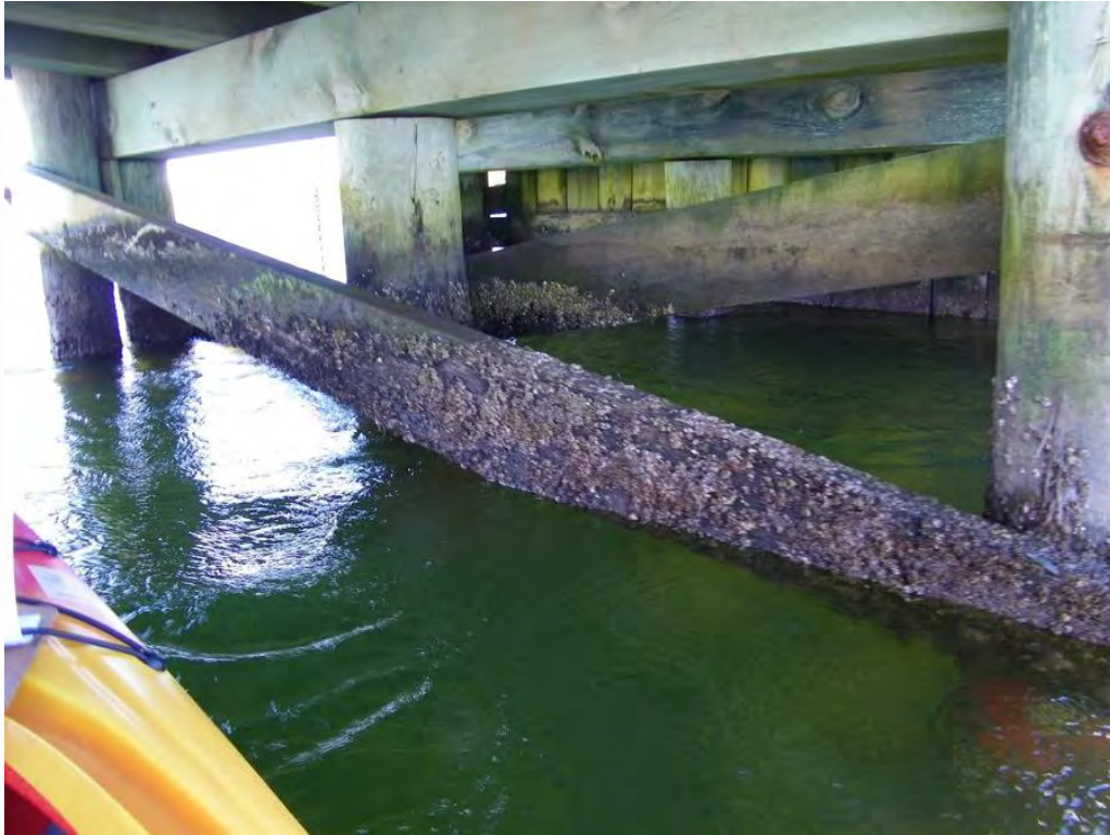
Photo 7: View pile bent 2, marine growth.
