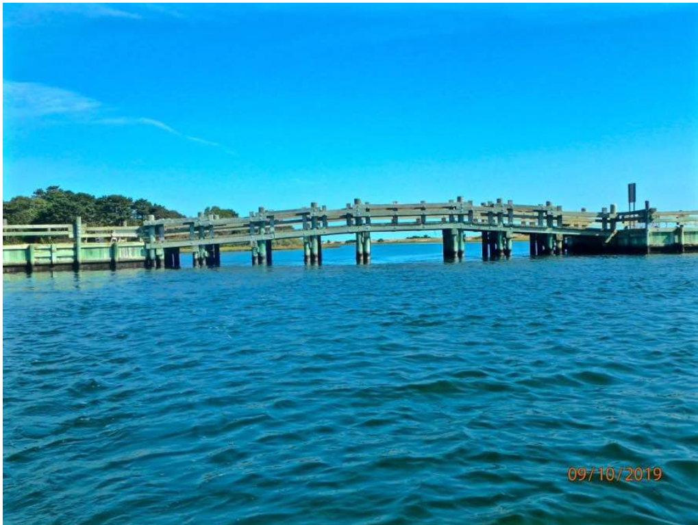
Photo 12: South elevation, typical vertical alignment of spans
