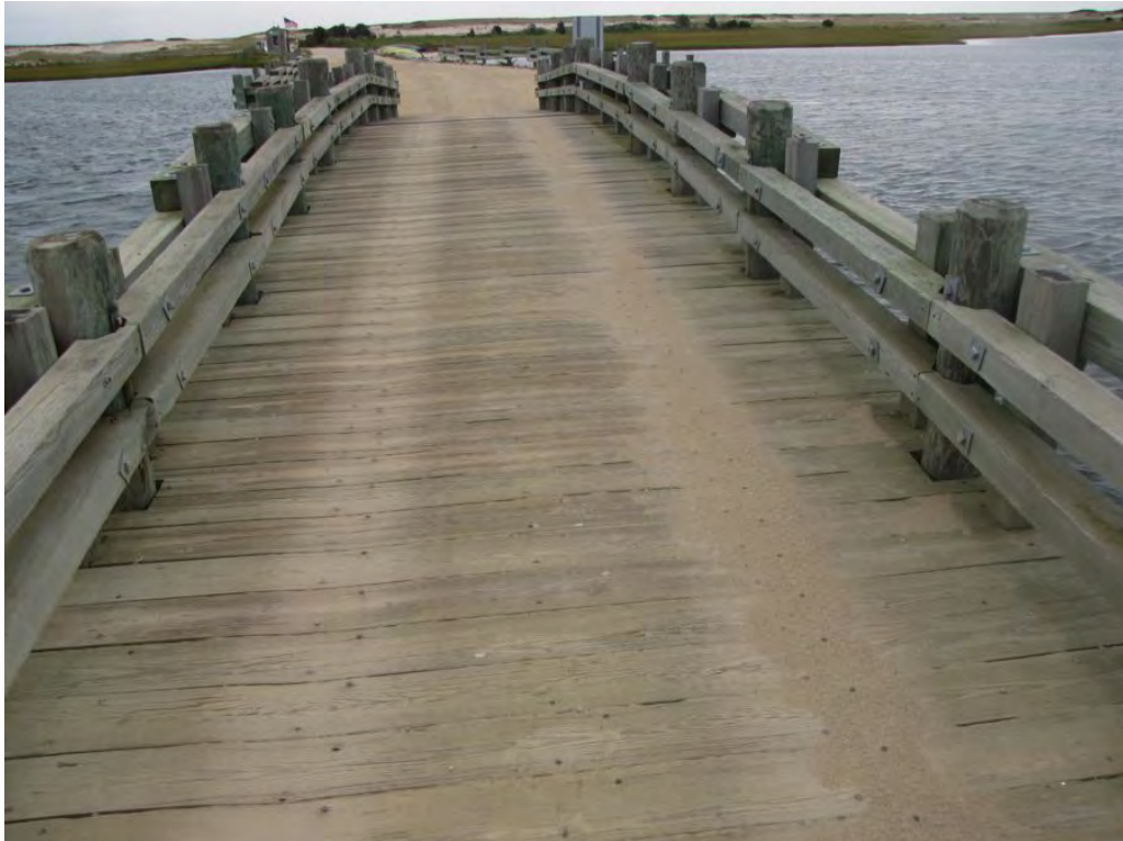
Photo 1: General topside looking east
