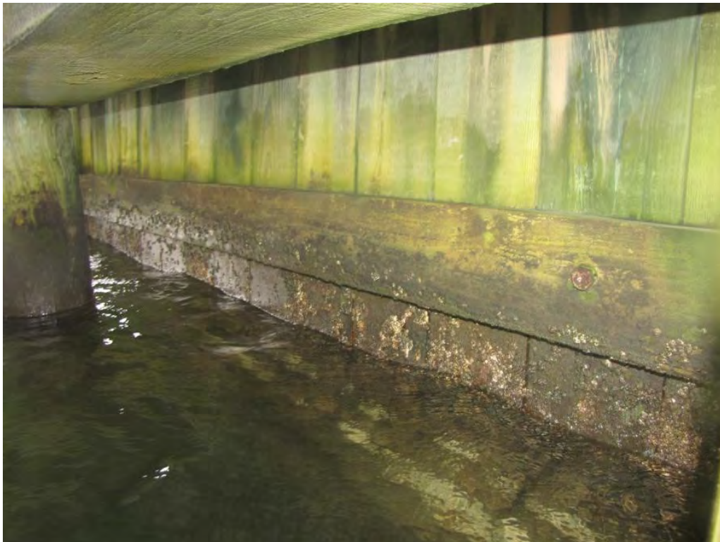
Photo 14: Typical pile and bulkhead along abutments
