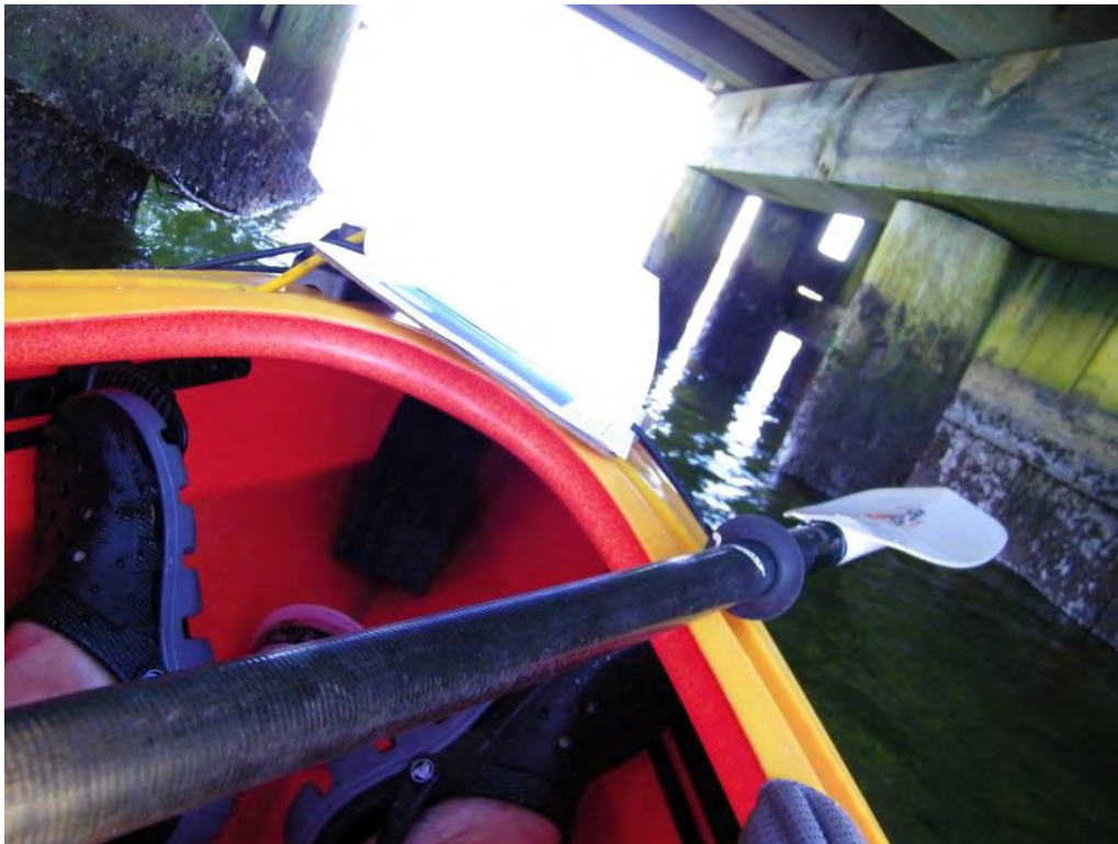
Photo 6: View pile bent 1 at west abutment.
