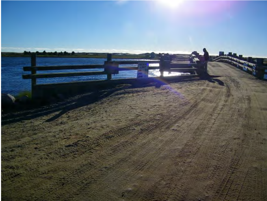
Photo 1: West at bridge posting sign.
