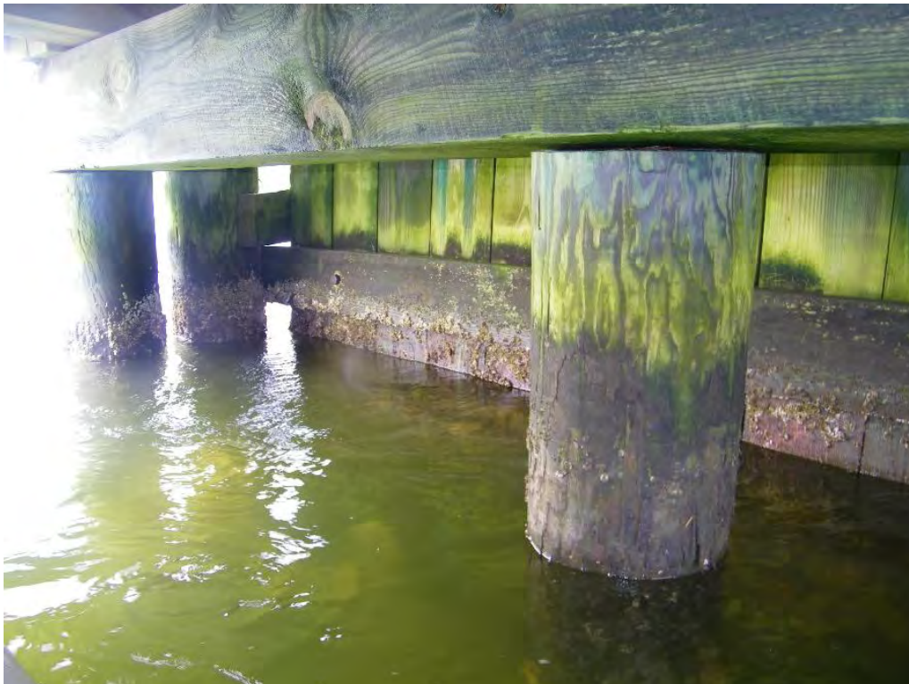
Photo 6: View pile/bent #1 @ west abut.
