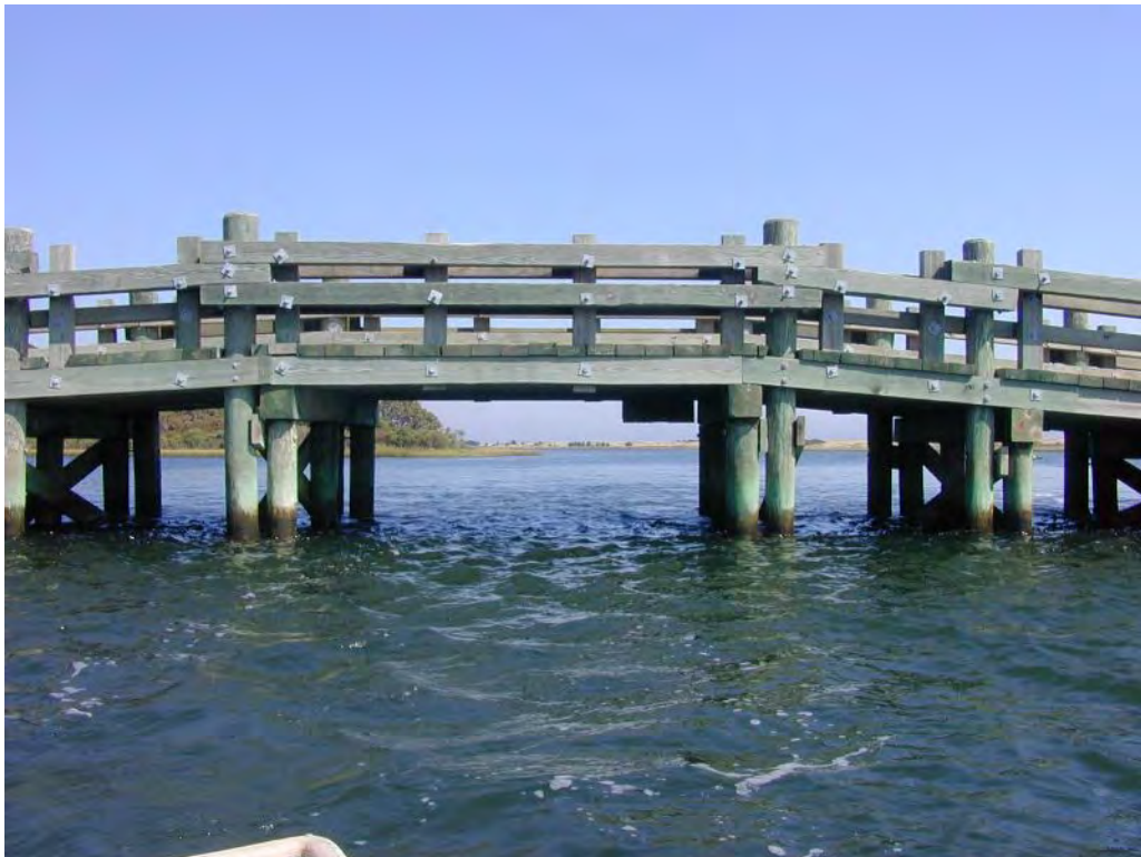
Photo 2: North view of main span.
