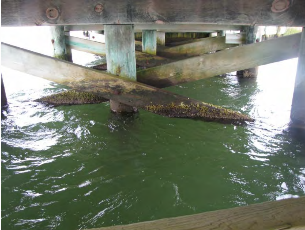
Photo 17: Typical overview of pile bents and diagonal bracing
