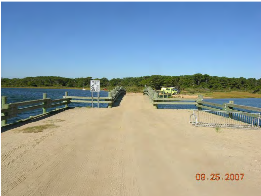
Photo 2: East approach showing weight posting sign on left
