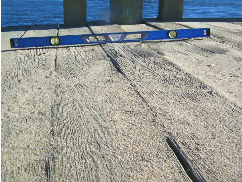
Photo 11: Common 1" spacings between top of nail heads and wheel rutting wear.
