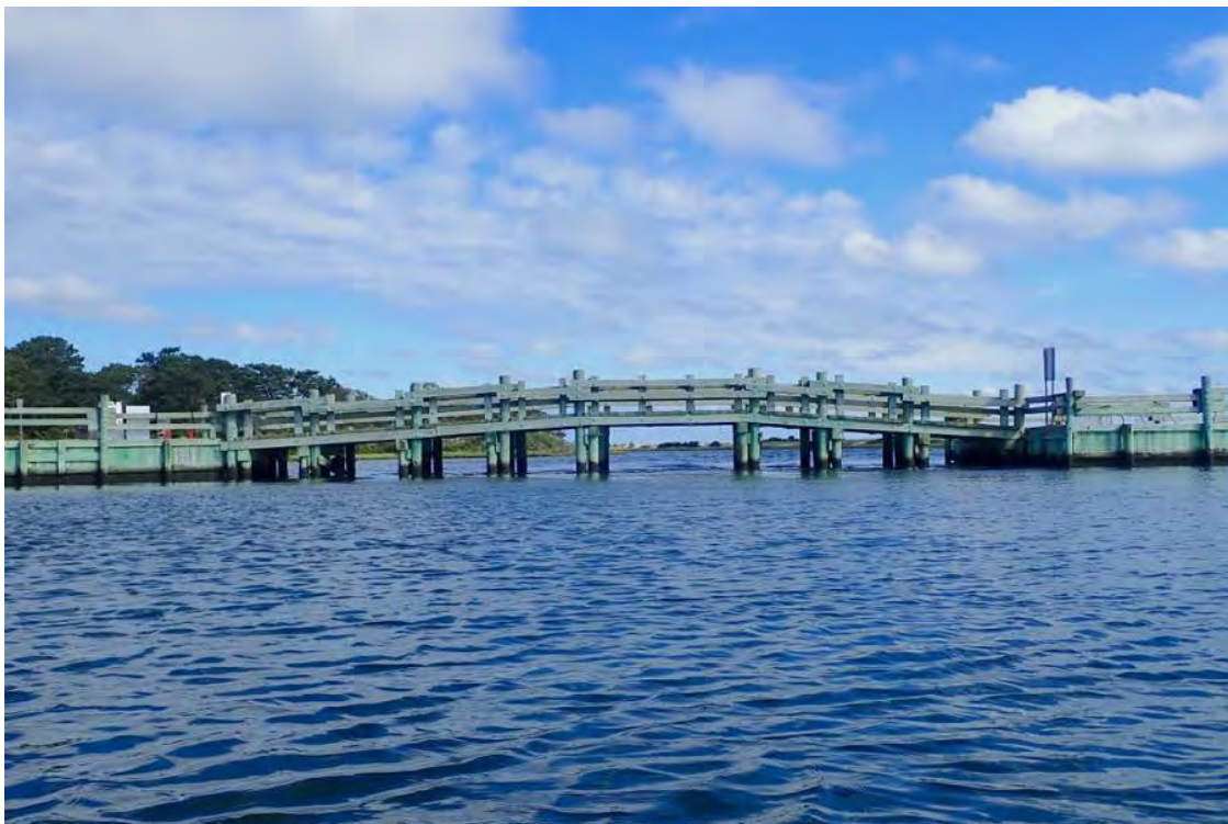
Photo 12: South elevation, typical vertical alignment of spans.
