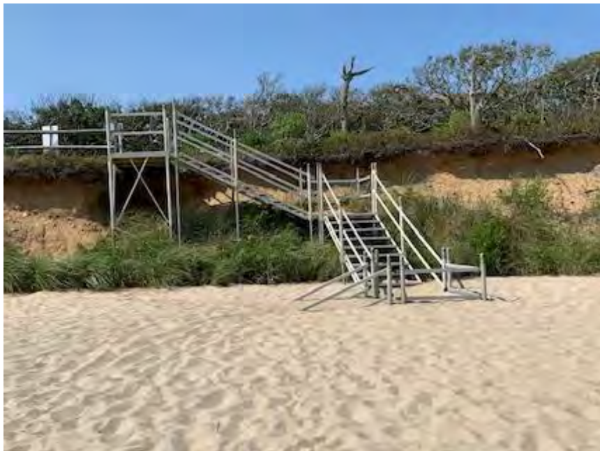
Figure 5: Modular stairs at Wasque Reservation
