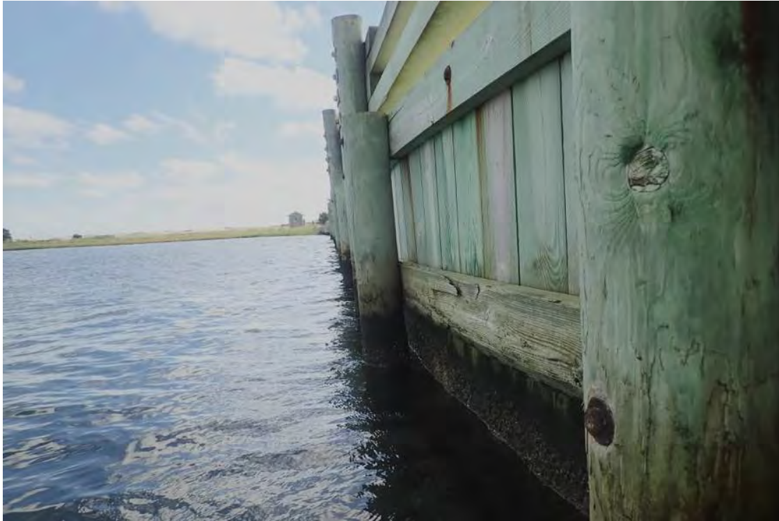
Photo 15: Northeast wingwall bulkhead between 1st & 2nd piles from west, split in middle wale.
