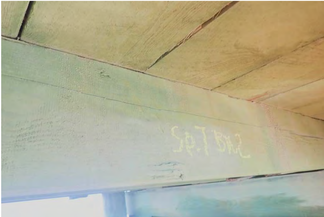
Photo 11: Span 7 Beam 2 south face, horizontal surface checking.
