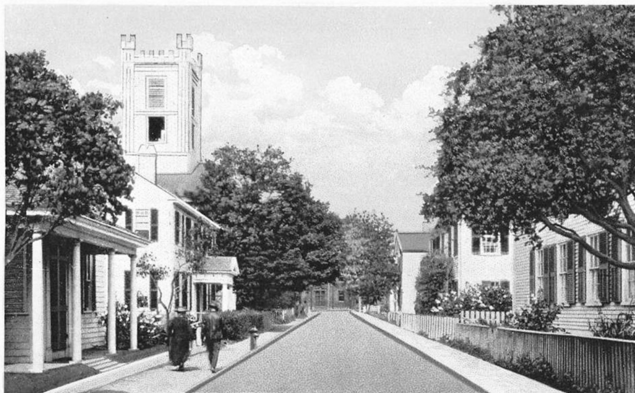
COFFIN HOUSE AND TOWER OF BAPTIST CHURCH, SCHOOL STREET, EDGARTOWN, MASS.
