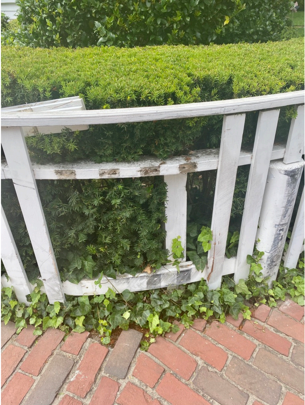
Whoops! Another bus didn't make it: corner of Pease's Point Way N. and Upper Main Street
