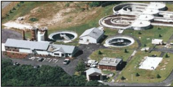
Figure 1: Wastewater Treatment Plant
